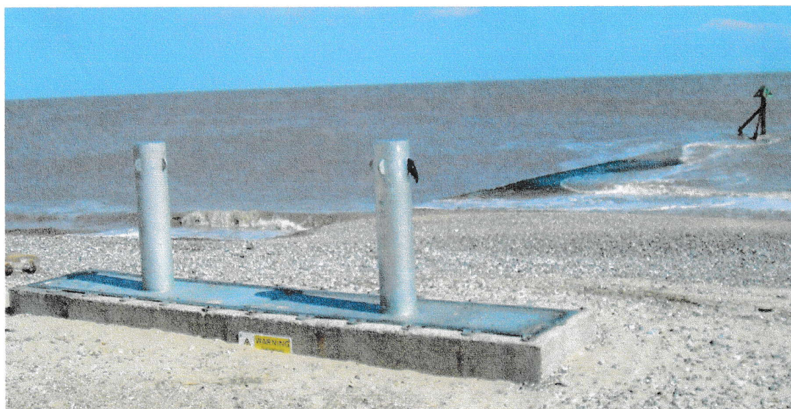
New air vents on sluice
