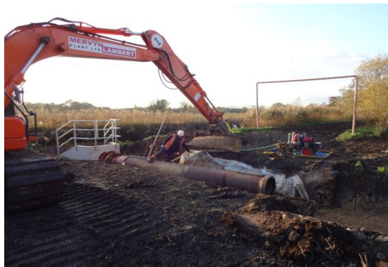
Figure 7 new sluice at Dam Bridge
