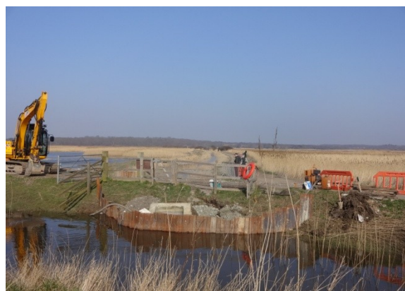
Figure 8 repairing sluice from RSPB reserve
