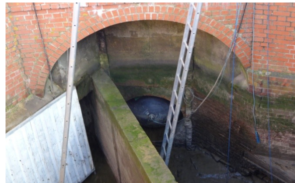
Figure 4 work on the sluice towards the sea.
