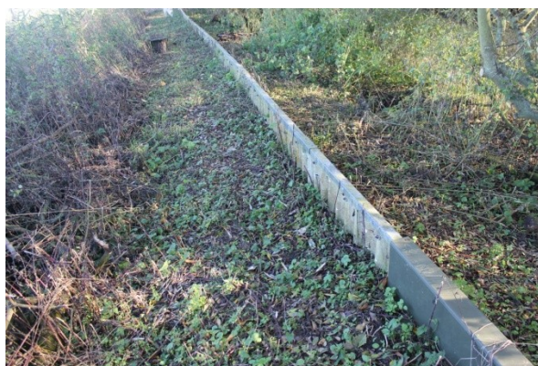
Figure 10 repair of exposed asbestos
