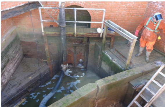
Figure 3 work on the Leiston Drain
