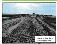
The footprint of an improved Coney Hill Cross Bank (North Wall) is in place. The placing of material and profiling of the new bank is expected to finish before the end of September. The construction of a new flow control structure will start soon, involving the laying of a new culvert, the installation of an outfall and the construction of an intake structure.
