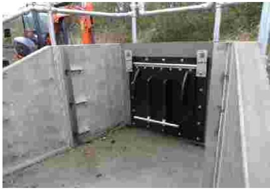
New Mumberry 2 sluice gate
