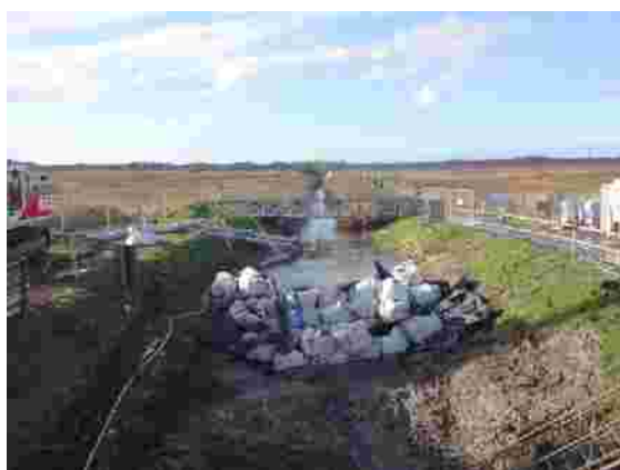
View up the New Cut with ballast bag dam
