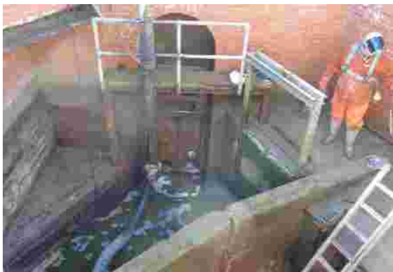
Inside sluice chamber towards Leiston drain
