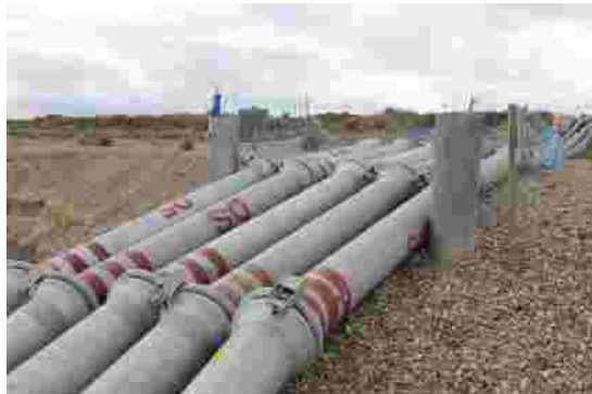
5 discharge tubes over the sea bank
