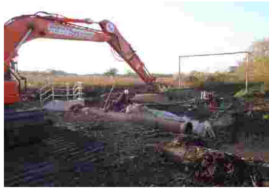
New Mumberry 2 sluice being laid in position.
