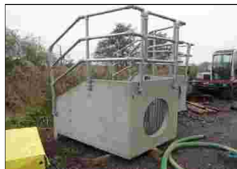
New Mumberry 2 sluice entry trap.
