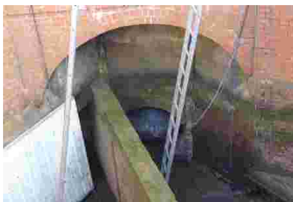
View inside sluice chamber towards sea
