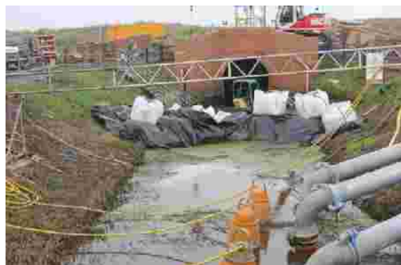
New Cut finally blocked with crane bag dam
